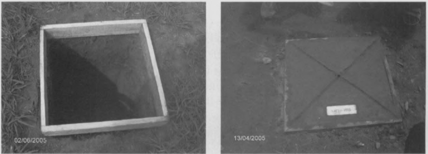
Fig. 3. — Pillar with identification label and centring point.
