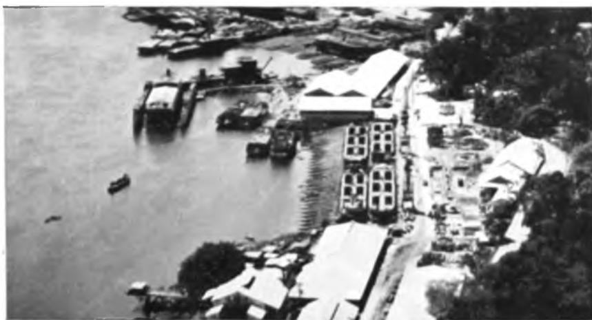
10. Chantier de remontage. (Cliché Chanic).
