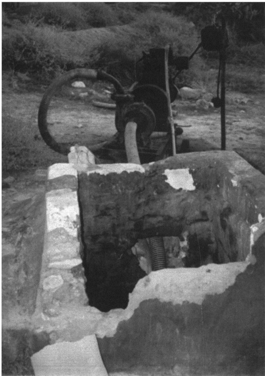
Fig. 1. — Roman water reservoir in Alexandria, Egypt, where (over)pumping resulted in complete drying-out of the reservoir.
