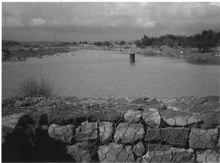
Fig. 3. — Recharge well and gabion dam in southern Tunisia.
