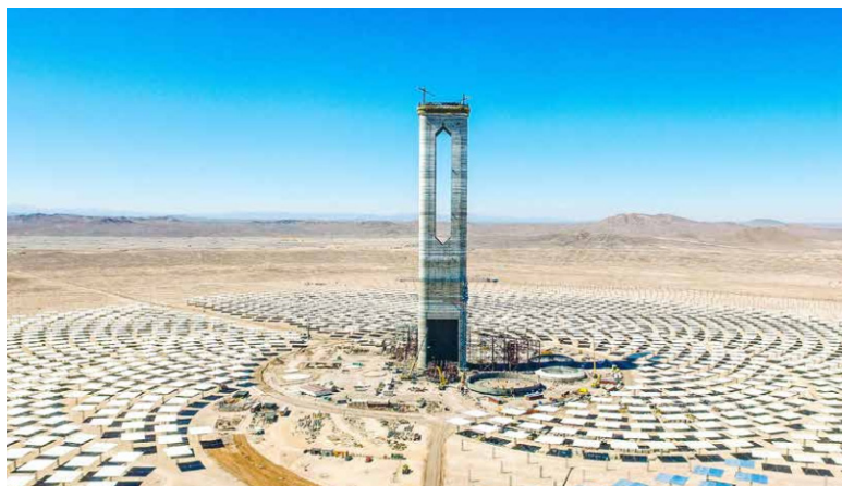
Fig. 4. — Atacama I power station under construction.
