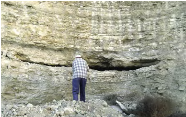
Fig. 17. — La Loteta dam: evidence of dissolution and subsidence observed in the gypsum unit during the excavation of the dam foundation (GUTIÉRREZ et al. 2015).
