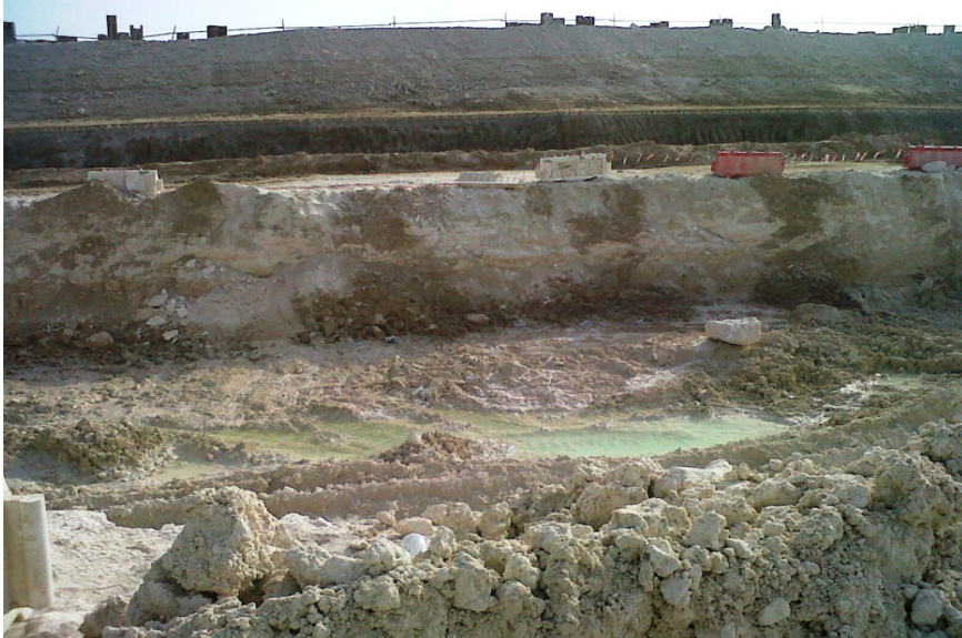
Fig. 14. — Above: excavation showing anhydrite interbedded in siltstone (Ruwais, UAE); below: veins and nodules included in hard clay matrix.
