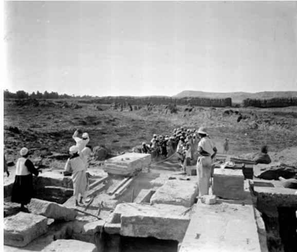
Fig. 6. — Excavations at Elkab, removal of a ceiling slab of crypt B in the temple of Nekhbet. Photo by Jean Capart, 5 March 1938 (© RMAH, inv. EGI 11477).
