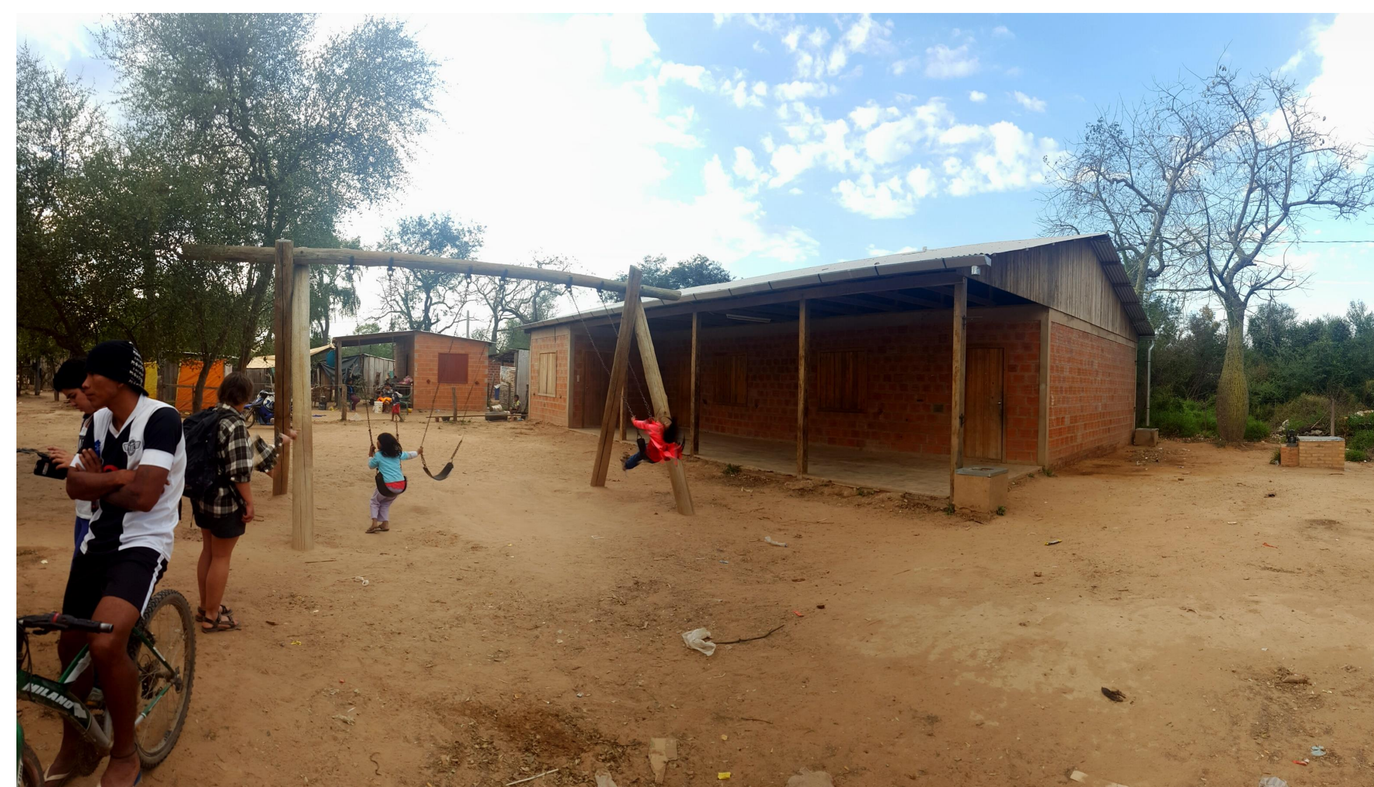
Informele nederzetting, Filadelfia, Chaco, Paraguay. Quartier informel, Filadelfia, Chaco, Paraguay.
