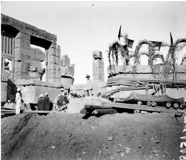
Fig. 10. Karnak, great hypostyle hall of the temple of Amun, restoration works by Georges Legrain. Photo by Jean Capart, 21 April 1909 (© RMAH, inv. EGI 1518).
