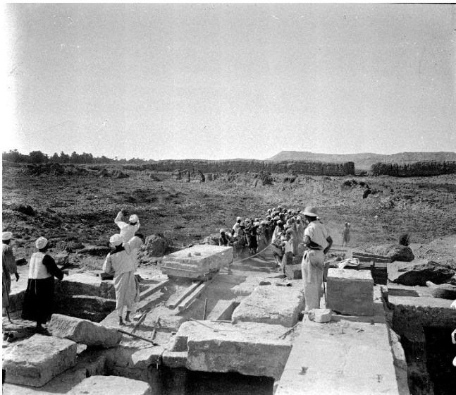
Fig. 6. Excavations at Elkab, removal of a ceiling slab of crypt B in the temple of Nekhbet. Photo by Jean Capart, 5 March 1938 (© RMAH, inv. EGI 11477).
